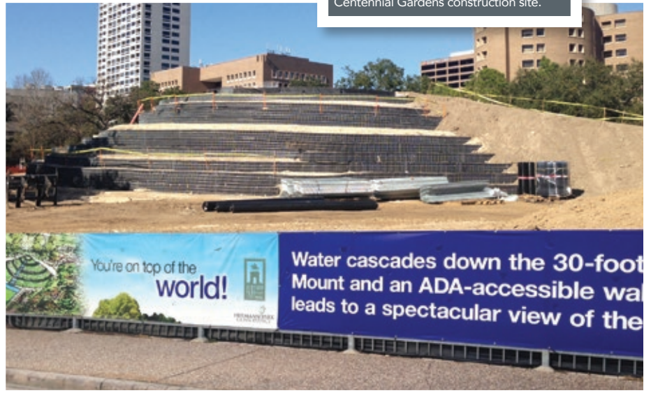
The garden mount rises at the McGovern Centennial Gardens construction site.
